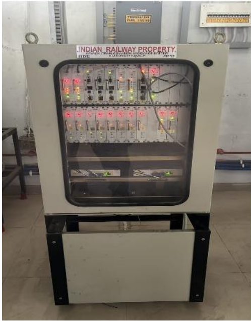
(Installation of Station Kavach)
