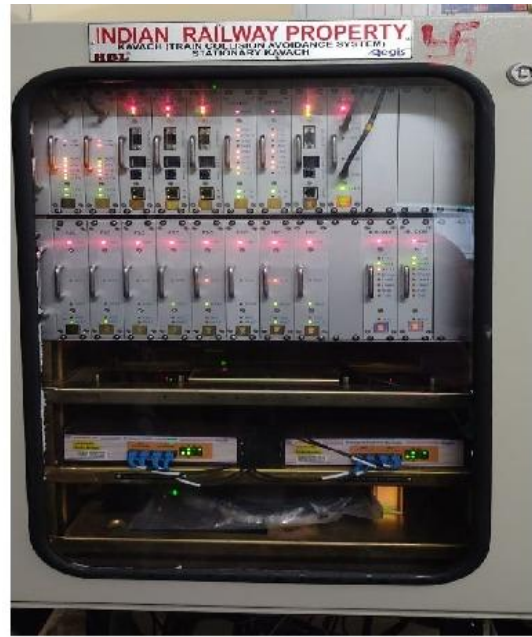
(Installation of Station Kavach)
