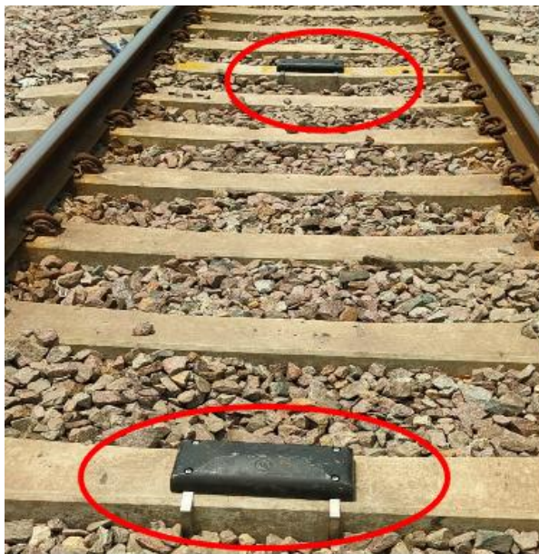
(Installation of RFID Tags on tracks)
