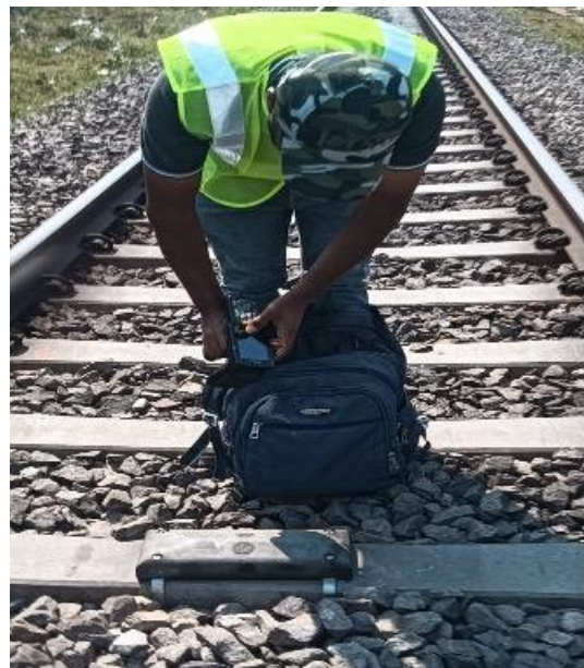
(Installation of RFID Tags on tracks)
